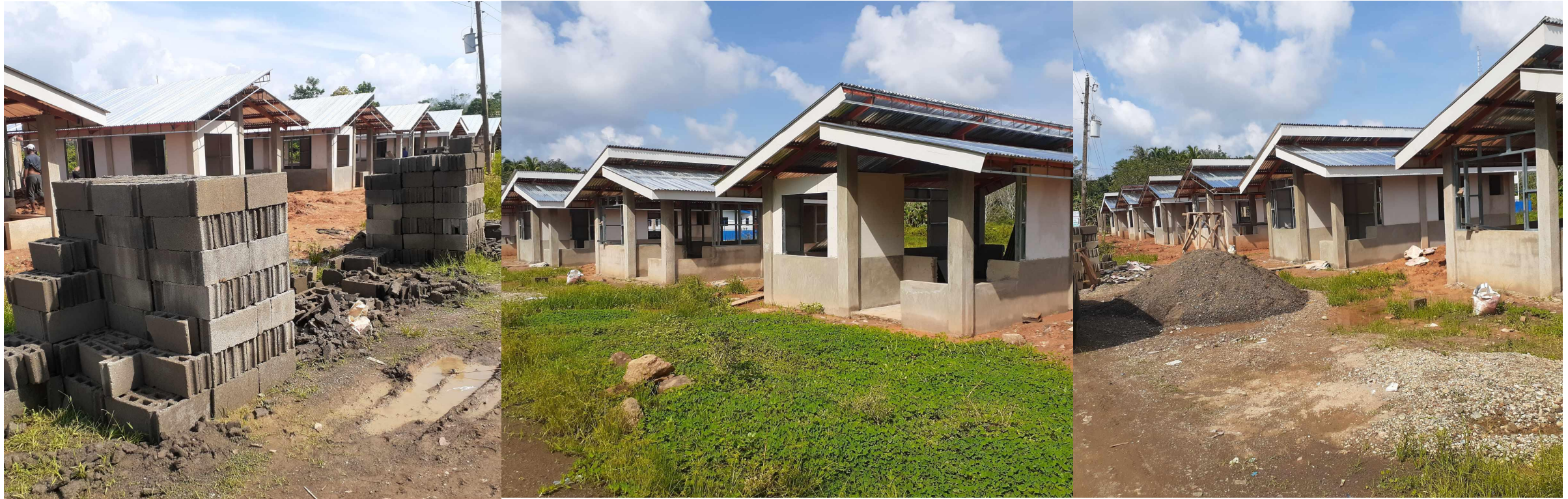
Datu Tumanggong Site Ongoing construction of 50 MSAP
