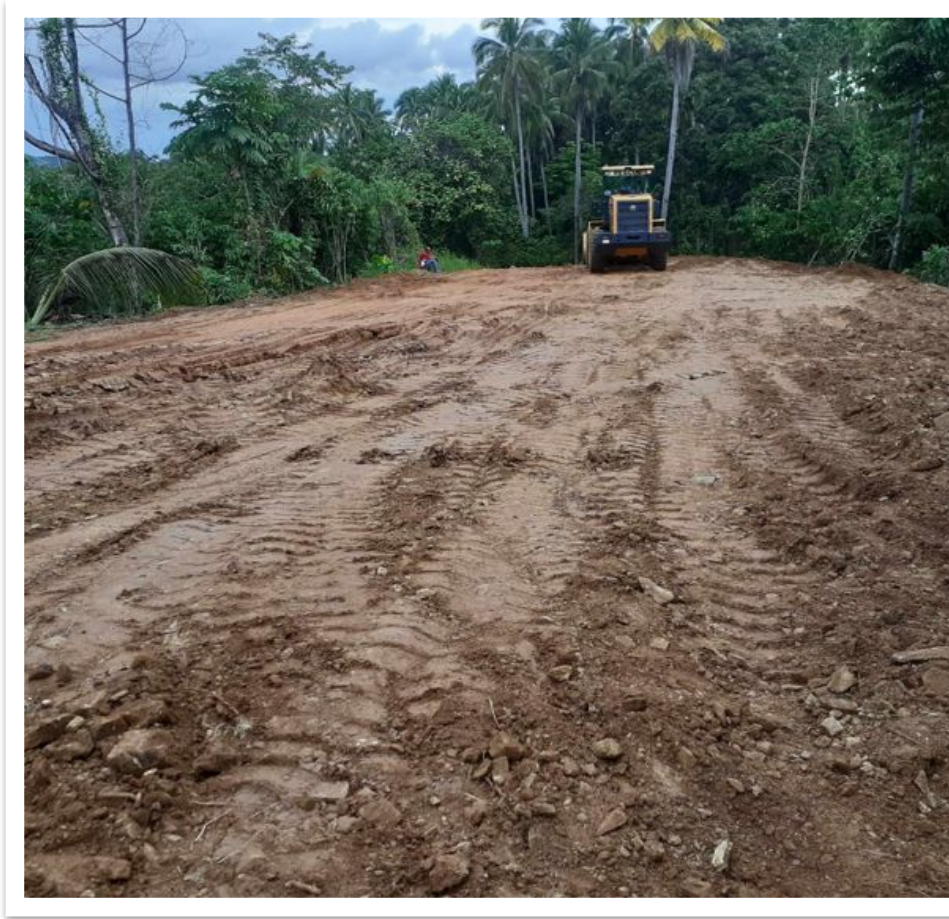
San Vicente Site Ongoing site development
